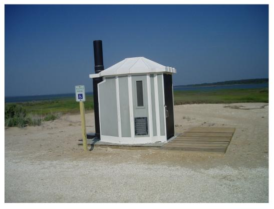
Moving from the planning stage to action, sustainable park infrastructure at Assateague Island NS was put in place. It was designed for a barrier island, where sea level rise and increase storm frequency are projected. This vault toilet mounted on a wooden deck allows easy relocation during storm events.
