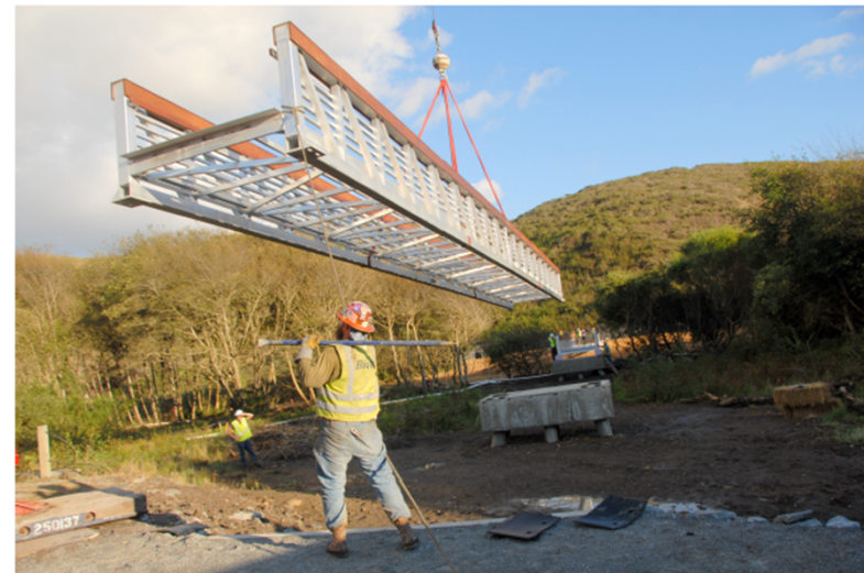
PEDESTRIAN BRIDGE INSTALLATION PHASE 3 2011
