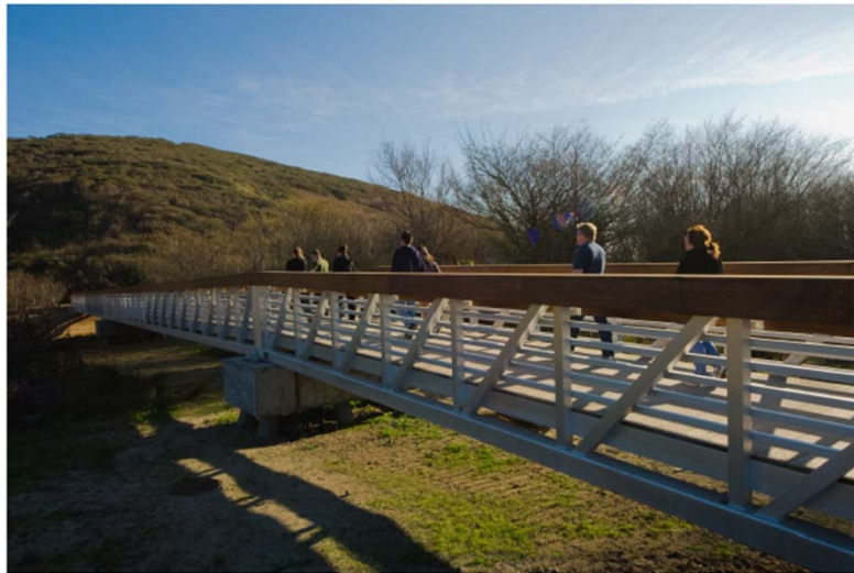
PEDESTRIAN BRIDGE INSTALLATION PHASE 3 2011
